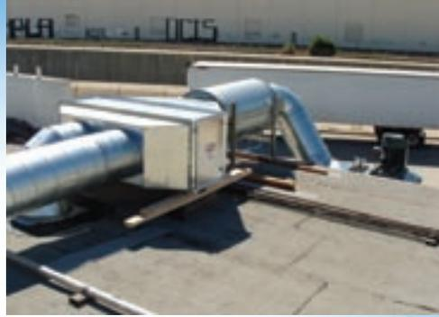
**Exhaust duct from the SFC downward flow dust collector with in-line silencer and safety filter.**
