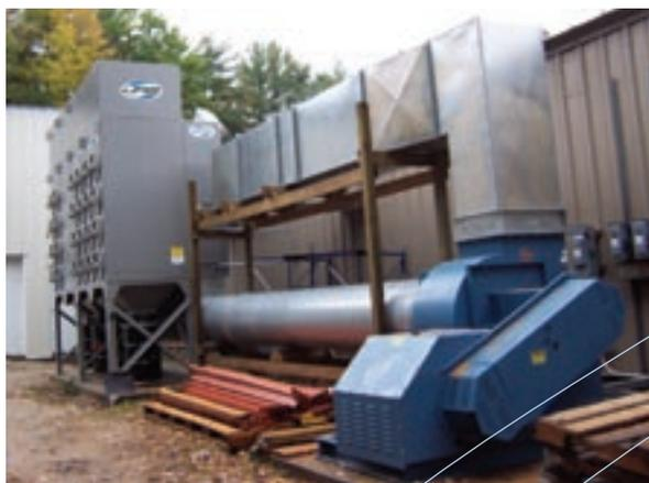
*A SFC 48-4 with an air distribution module and ground mount blower collects plastic dust.*
